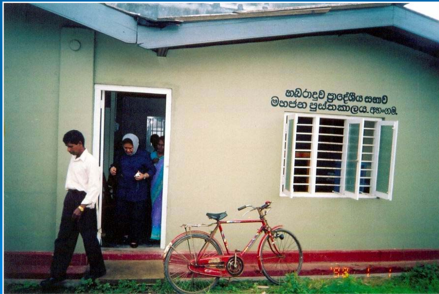
A recently repaired public library
